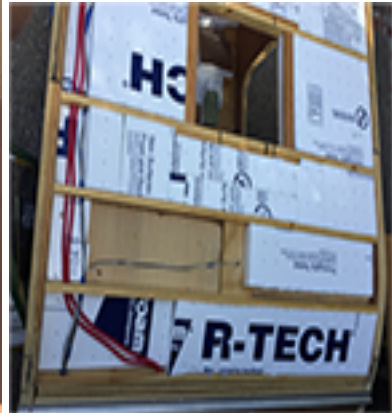
Roof – insulation + wiring
