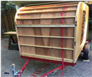
Red battery wires
