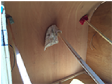
Applying pressure to the Luan curve
