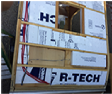
Wiring through ceiling spars
