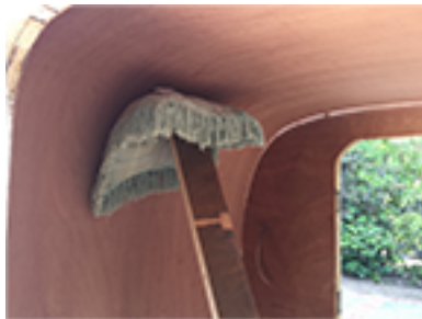
Applying pressure to the Luan curve
